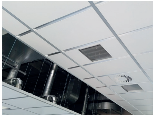
Detail of panel suspension
